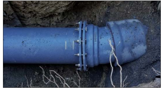
FIG. 11 An example of DN375 x 11 degree bend showing: 1. Type NS Mechanical Bend, Tee Bolts and Gland plate. 2. Type NS mechanical bend socket installed into Type NS Pipe Socket
