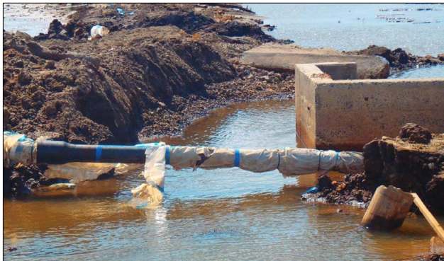
FIG. 9 SRDIP pipe remaining intact during the 2011 Japan Earthquake
