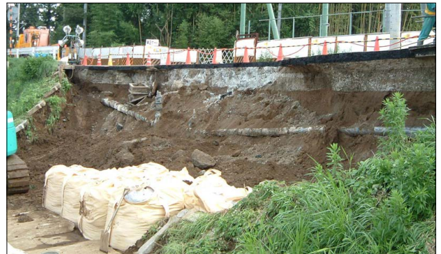
FIG. 10 SRDIP pipe remaining intact during the 2011 Japan Earthquake
