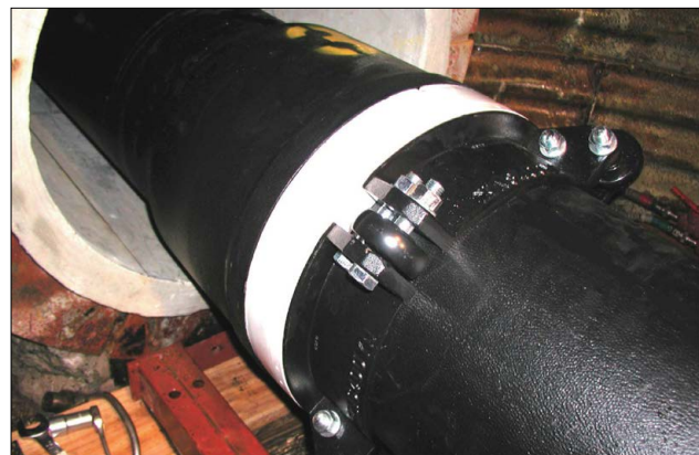
FIG. 18 Pipe casters set on the pipe barrel
