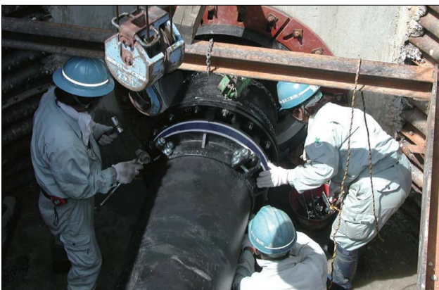
FIG. 17 Work In progress
