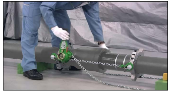
FIG. 12 Type NS pipe joint being made using special tools.
