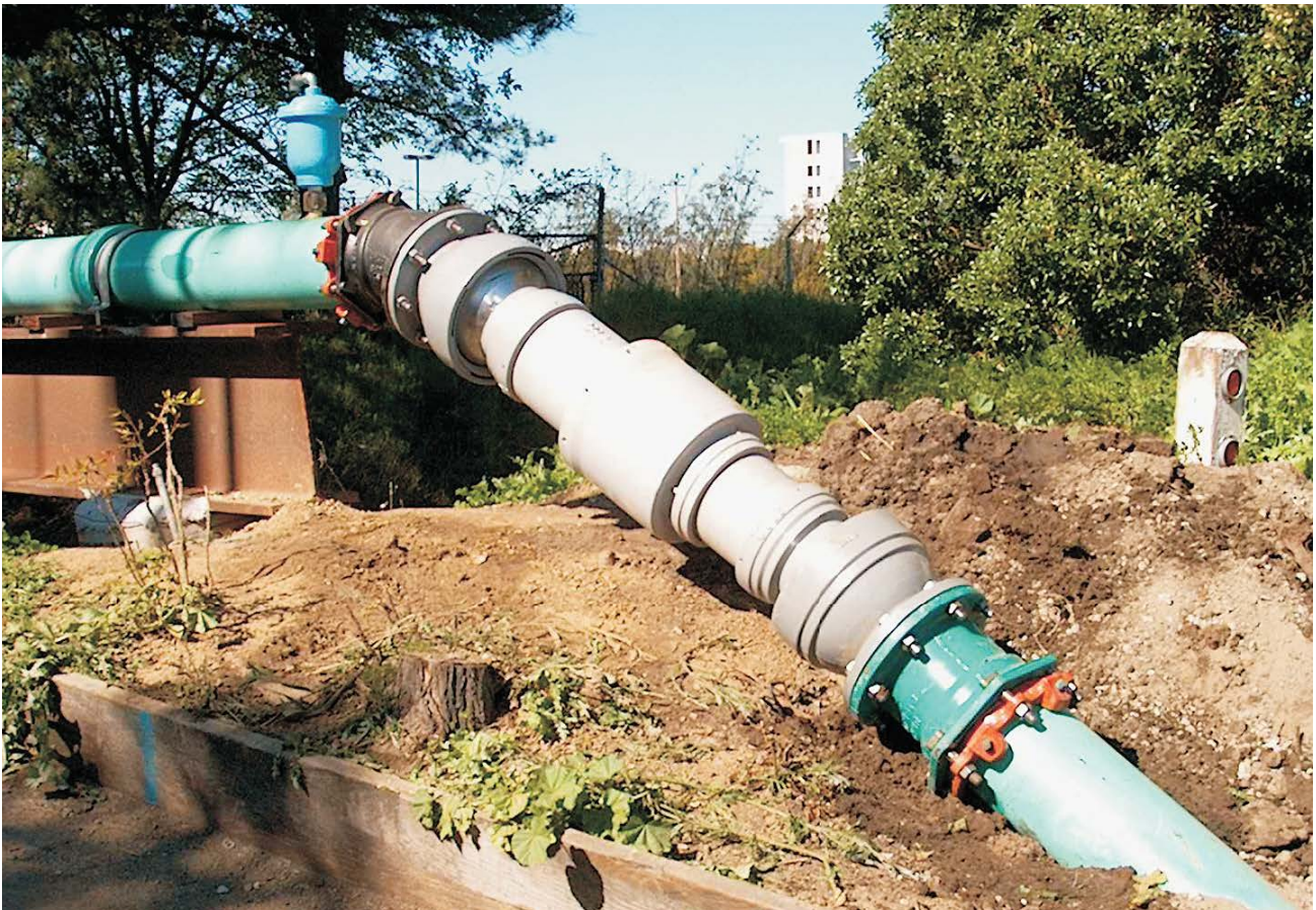
FIG. 1 DN200 Force Balanced Flex-Tend
